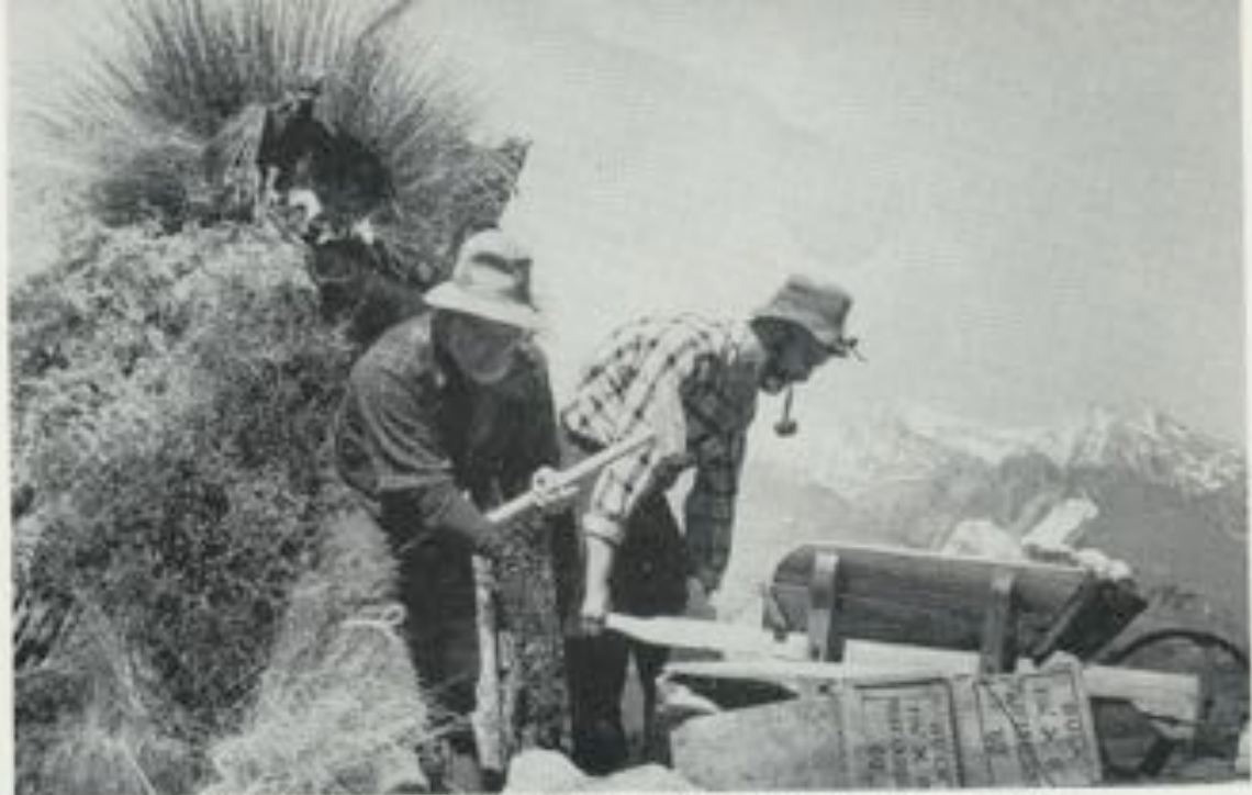
A demonstration of the original method of scheelite mining in the district, using 10 pound hammer and wheelbarrow.
